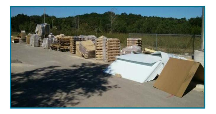
Cardboard material needed for the foundation was delivered on site and the following work were completed—Trenching for underground beams, Installing the cardboard, Binding the foundation steel over cardboard, and Engineering & City inspections—before pouring the concrete.
